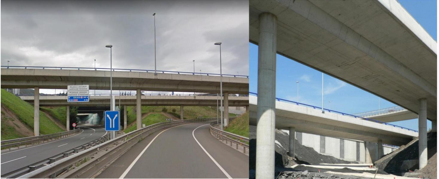
The reinforced hollow slabs cover a maximum span of 23.0m with maximum depths of 1.15m (L/20) and have been projected as bridges free of supports or expansion joints which therefore greatly reduce the maintenance costs. To do this, the circular shafts are embedded in the deck and the load beams and are founded on micro-piles.
